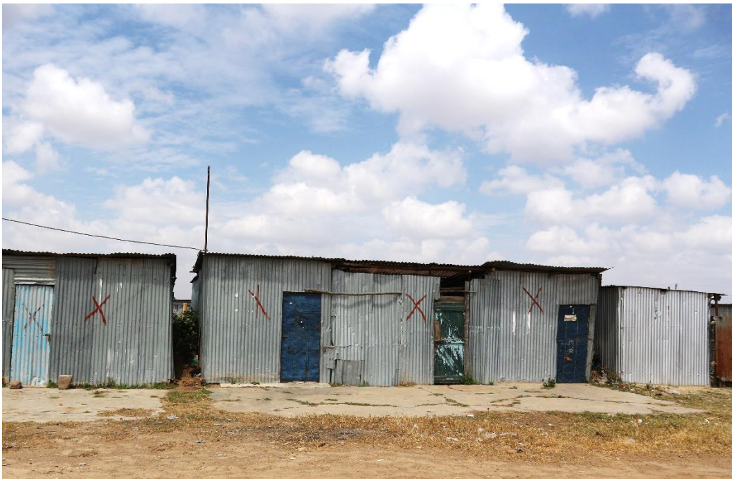
Figure 5.6 Structures with sign 'X' which will be demolished
