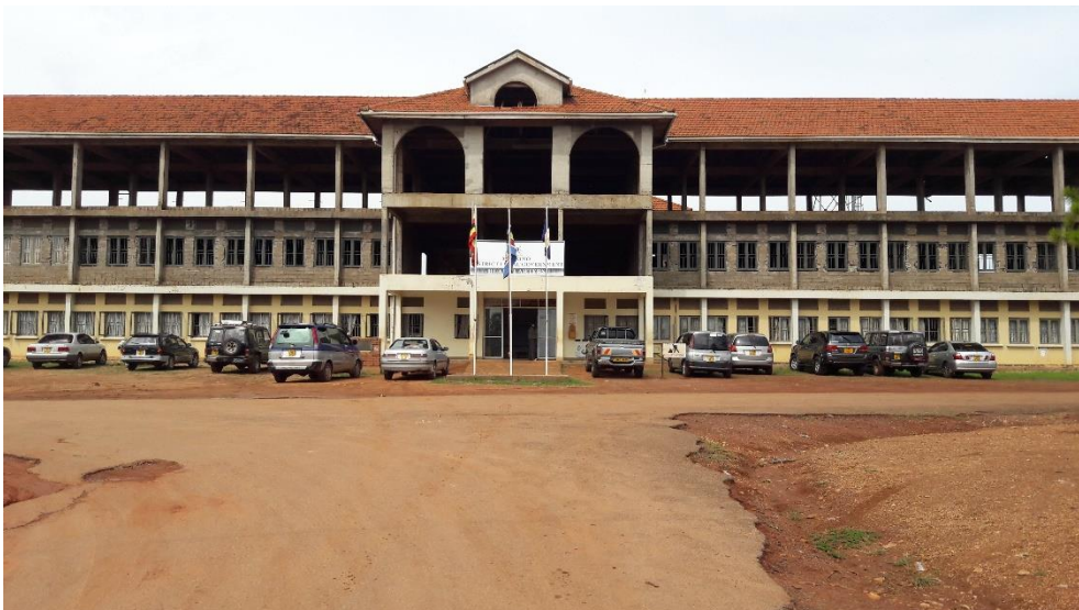
Figure 9: Mukono district local government office
