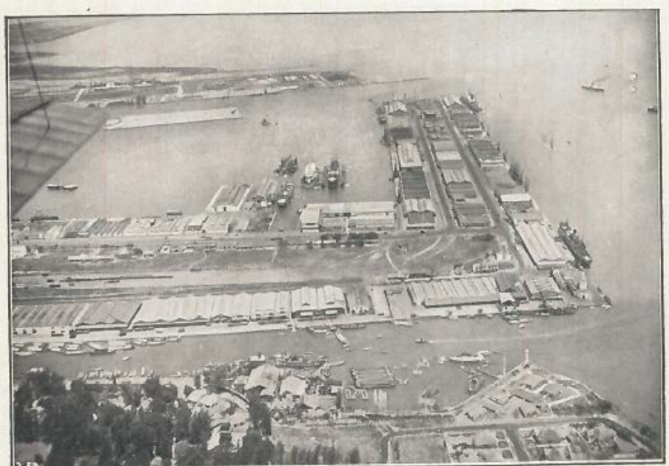
Airplane view of the harbourworks at Tandjong Priok.
