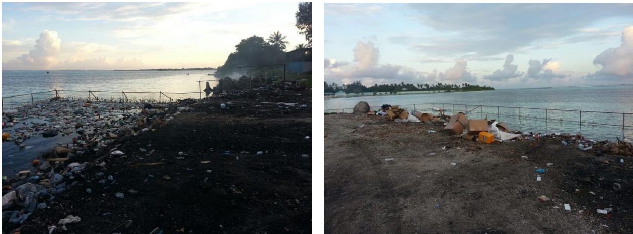
Figure 2-2 and 2-3: Reclamation of land on Himmafushi by using waste 26
