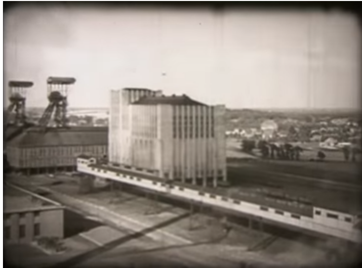
Figure 66: Aerial view of the plant.
