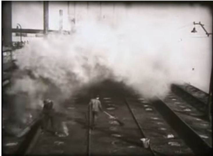
Figure 68: Workers seal the oven under harsh conditions.
