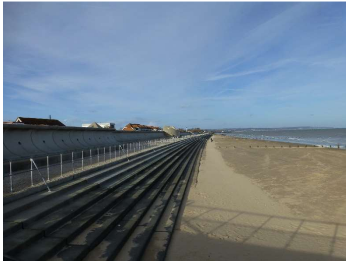
Dymchurch Seawall, Romney Marsh, UK (own photograph)
