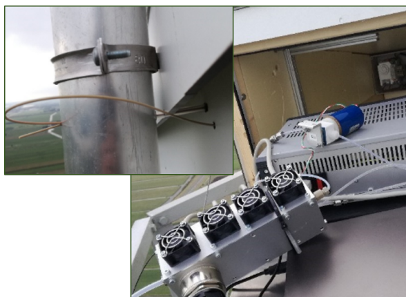
Figure 8: The flow controller (blue device) that provides a secondary access to the nitrogen is shown here. The nitrogen tube is placed in the sampling tube as shown in the expanded photo.
