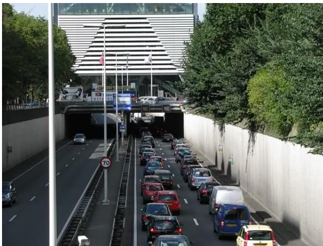
Figure 25 Building (Malietoren) above the Utrechtsebaan (A12) The Hague source:www.wegenforum.nl
