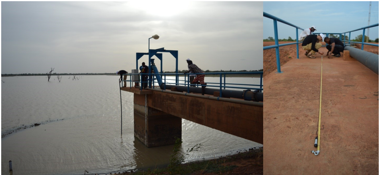
Figure 8: Installation of a diver. Photos taken on August 12, 2016 by F. van Broekhoven
