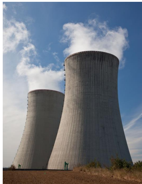
Figure 6: Typical cooling tower (ATS, 2017).
