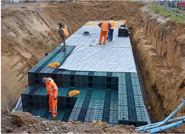
Figure 5.3: Infiltration structure that is built up from many separate infiltration boxes. Image copied from Indra, 2016.
