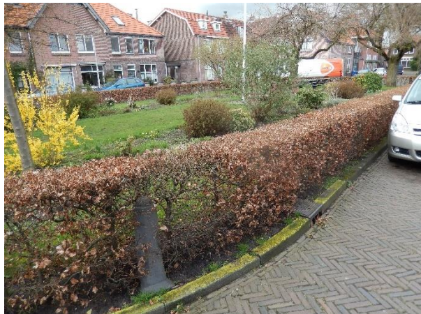
Figure 1.5: One of the green areas (Palmstraat) in the Soesterkwartier that is located above street level and is surrounded by curbs. Rainwater that falls on the street enters the sewer system instead of runoff to the green areas.
