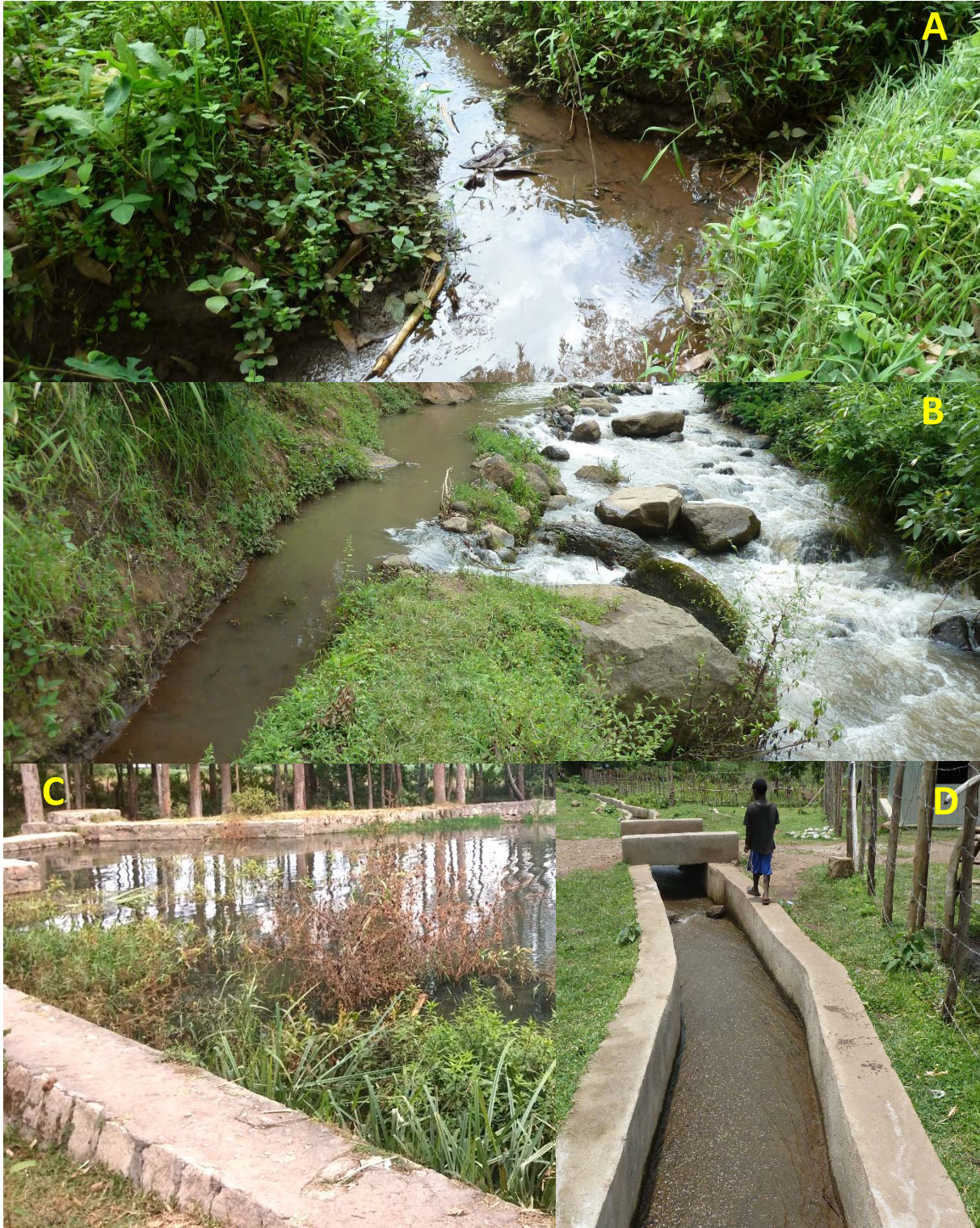
Figure 4: Different irrigation structures in the Tikur Woha subbasin: A small and dense irrigation network between agricultural plots, B a one meter width irrigation channel diverts water from the Wosha stream to the crops nearby, C artificial reservoir filled with water for irrigation purposes and D this concrete irrigation channel is built recently.
