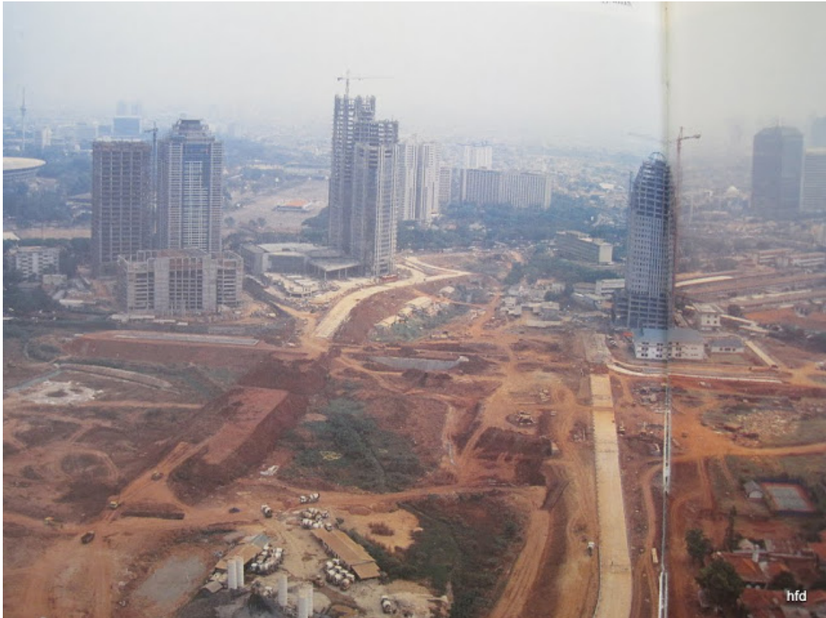
Fig. 4.5. Closed down construction projects in Jakarta, ca. 1995.
