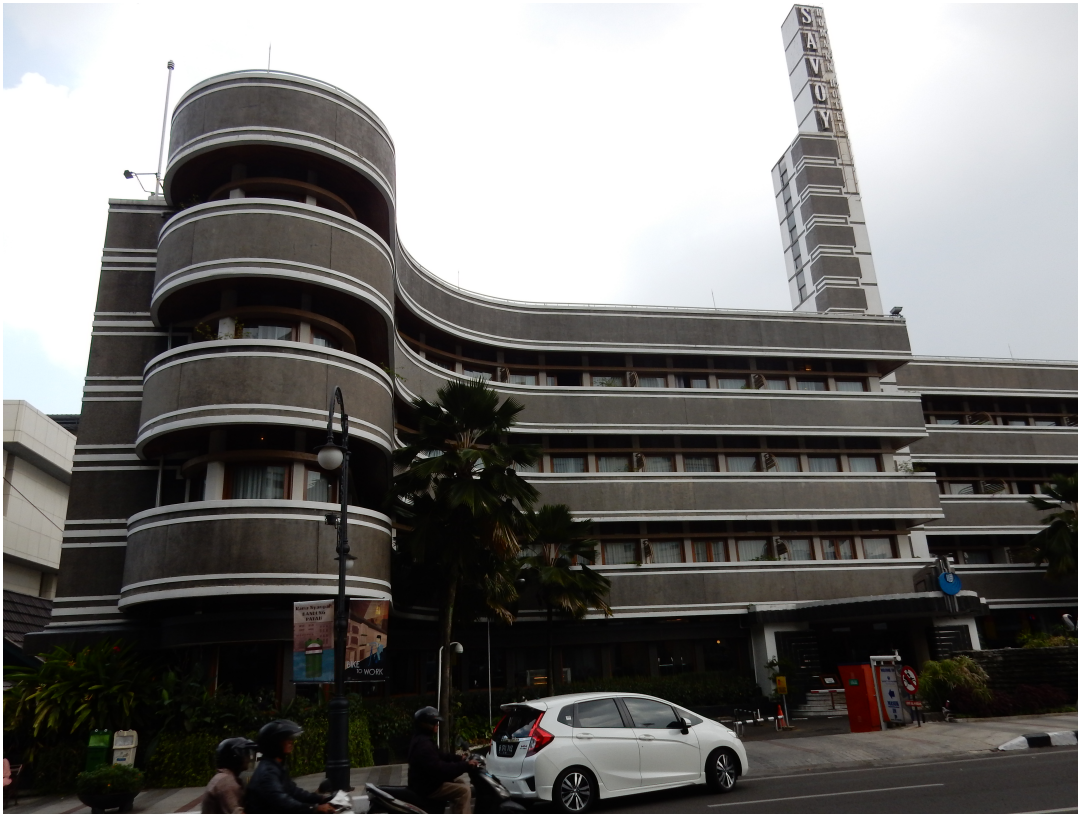
Fig. 5.12. Hotel Savoy Homann. Built in 1939 by A. Aalbers. It reflects a Modernistic style with Art Deco elements, with its curved streamlined forms.
