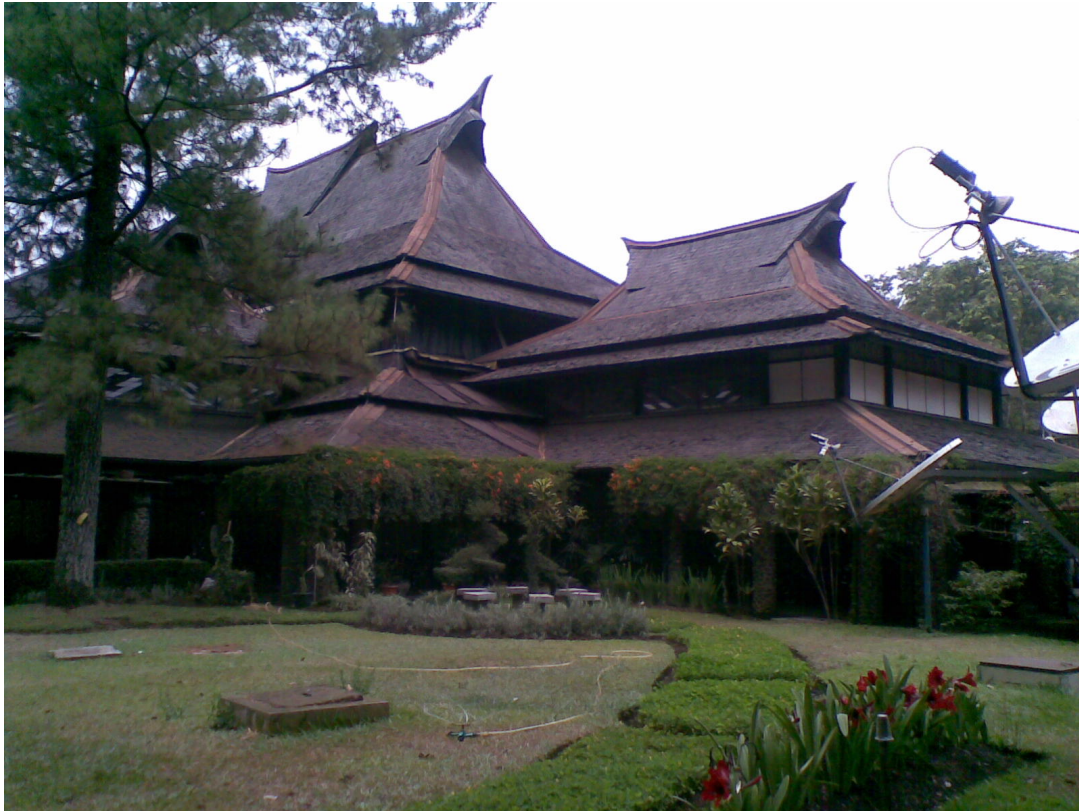
Fig. 5.14. Auditorium of ITB. Built in 1920 by H. Maclaine Pont. Especially the roofs reflect indigenous building constructions from Sumatran architecture. In the interior Maclaine Pont used arch trusses developed by the French engineer A. Emy.
