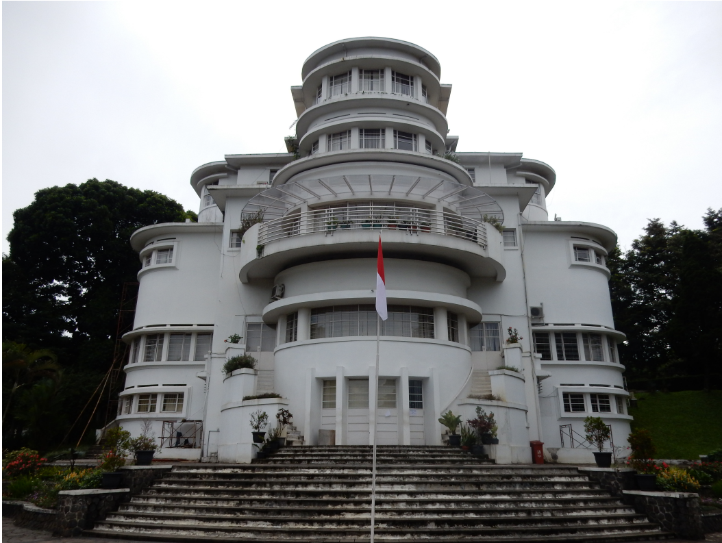
Fig. 5.10. Villa Isola. Built in 1932-1933 by C.P. Wolff Schoemaker. Built as a residential house for a famous Dutch media tycoon. Currently in function as the headmastership office of the University of Education (UPI).
