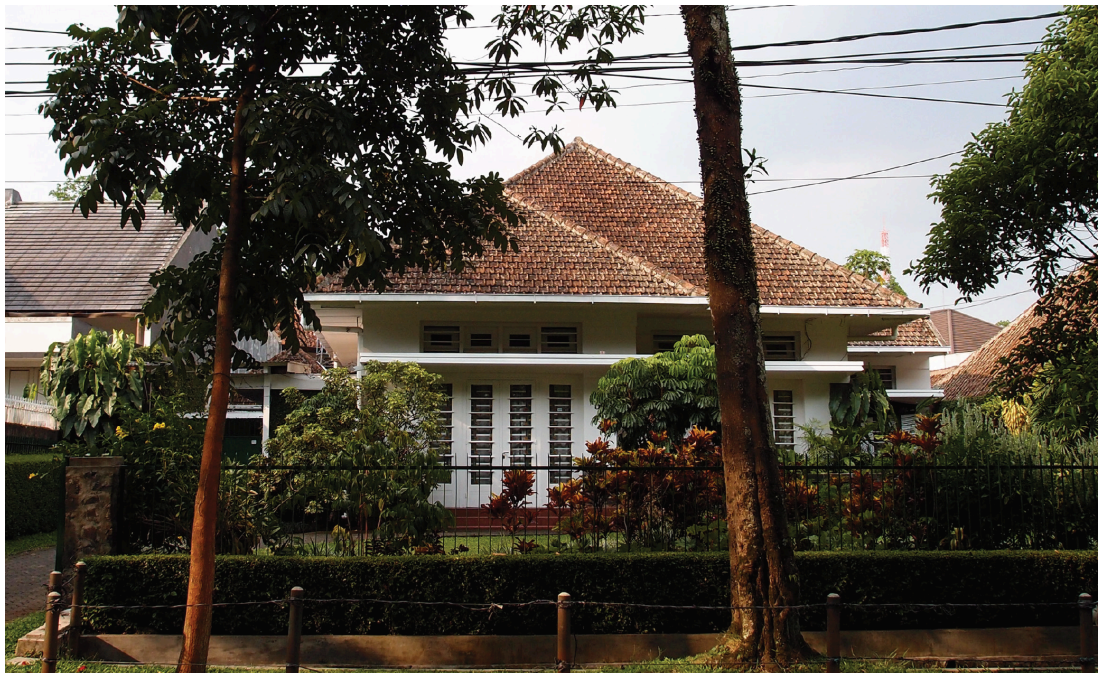
Fig. 5.15. Villa type residential house, ca. 1920-1930.
