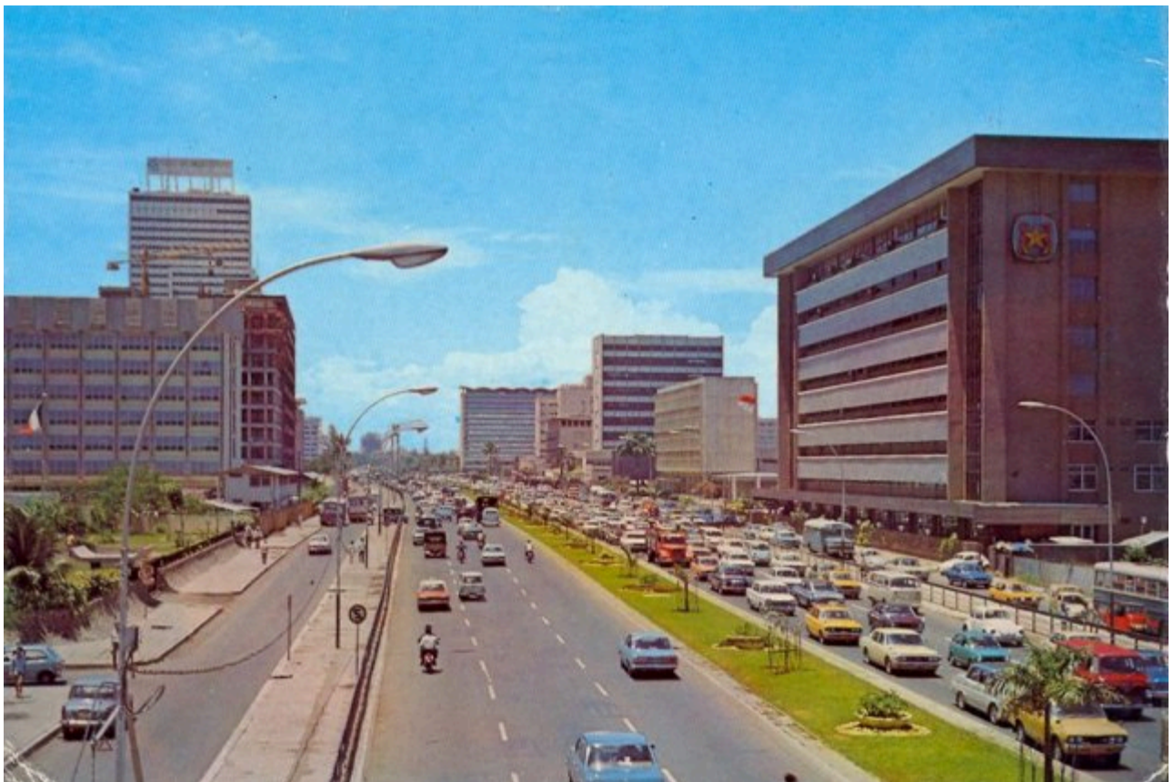
Fig. 4.2. Thamrin Street, Jakarta, one of the most important thoroughfares, along which iconic high-rise buildings were erected, ca. 1975.
