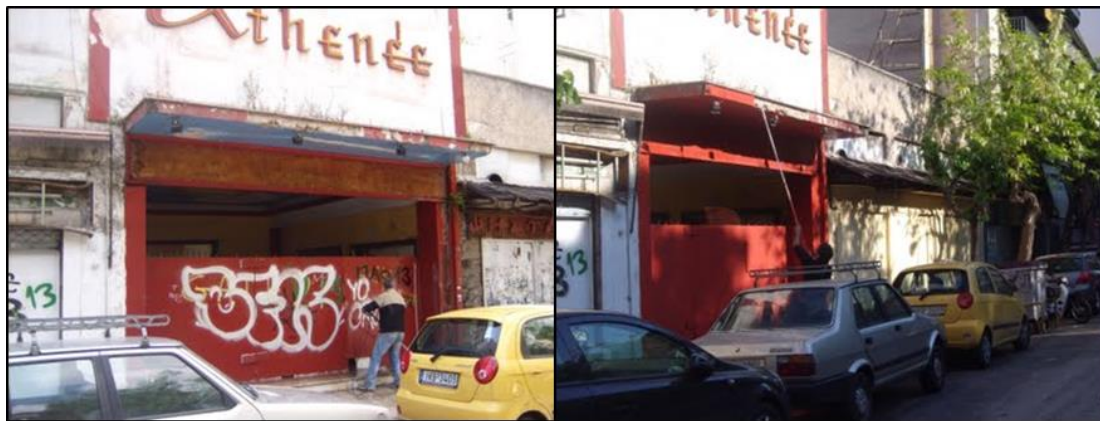
Picture 33. The Before and After the intervention at Attene cinema
