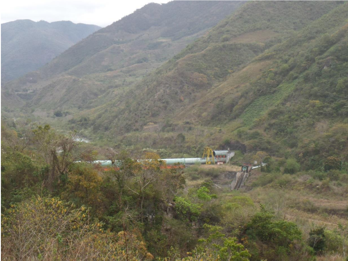
Photograph 7. The tunnel constructed by INDE, close to Agua Blanca. This photograph was taken on 06-03-16 during our first visit to the community.
