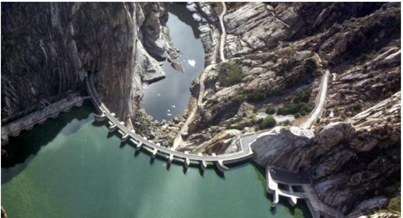
Aldeadavila dam, Spain. Source: www.rechargenews.com
