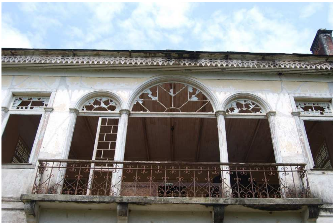
Fig. 7. Roça Boa Entrada, detail 1st floor. Note the thin fluted cast-iron door posts, the stained glass motives, cast iron fencing, and the fretwork capping the roof, 2012.
