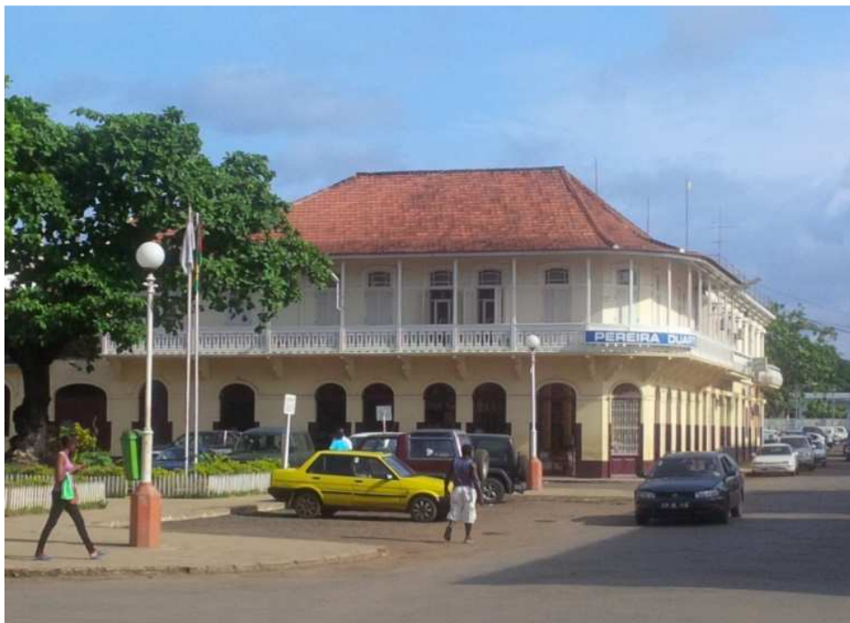
Fig. 33. Large residence with shops at ground floor level in central São Tomé town, 2015. Of note are the large veranda, ornate balcony railing, louvered entrance doors & louver shutters.
