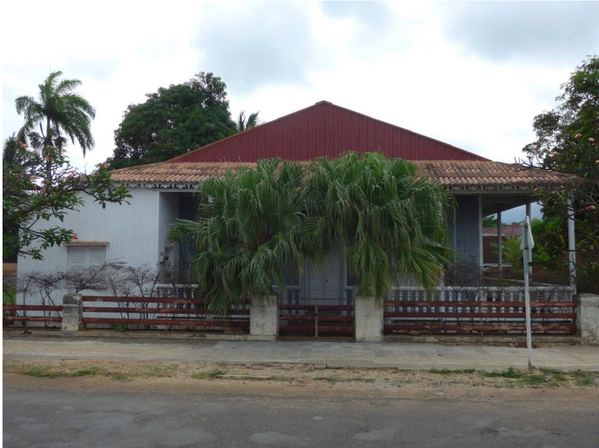
Fig 113. Facade of the 3 rd surviving sea fronting workers cottage, substantially altered, 2015.
