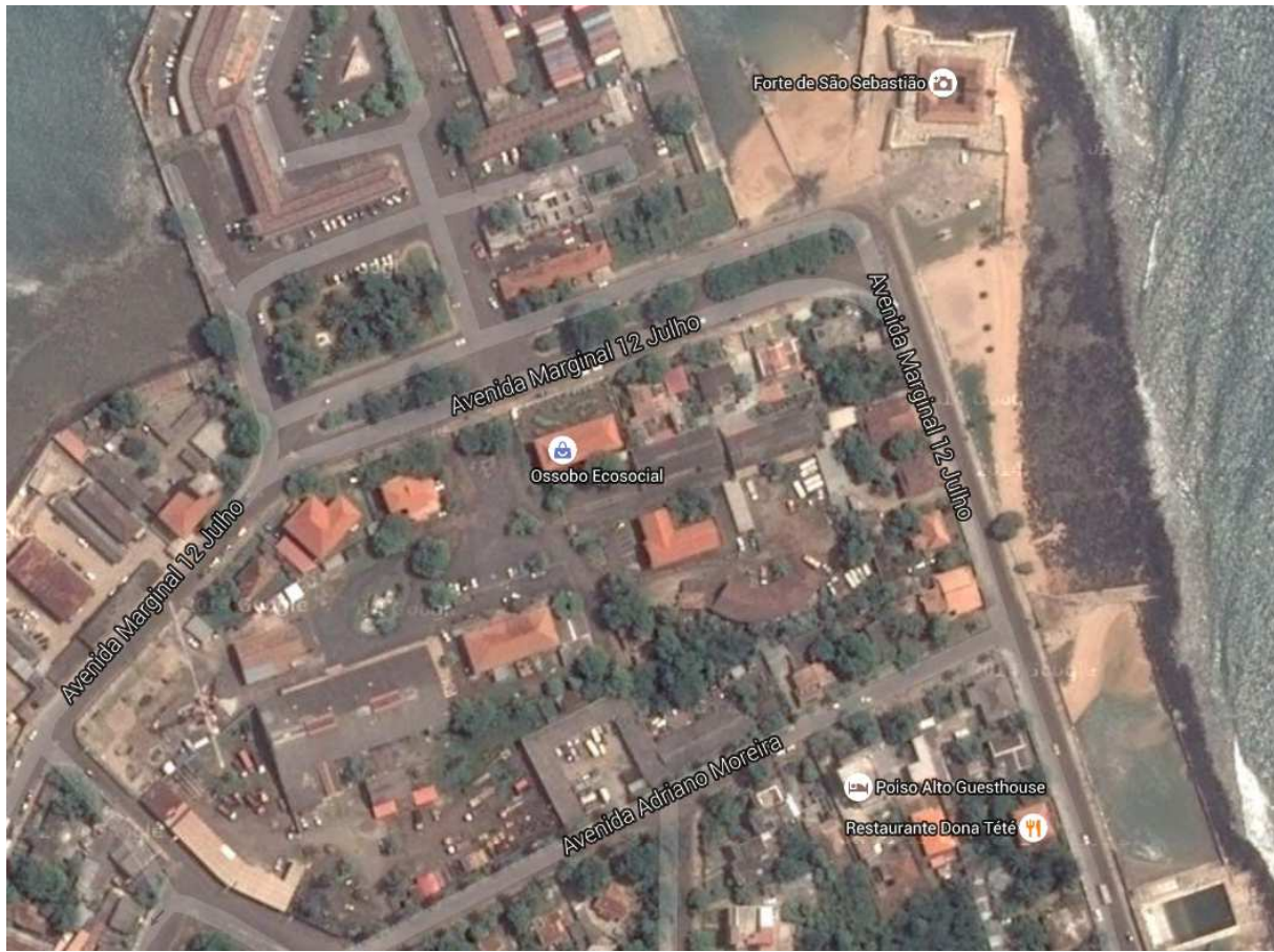
Fig. 100. Aerial view of the S. Sebastião Maritime Station circa 2010.
