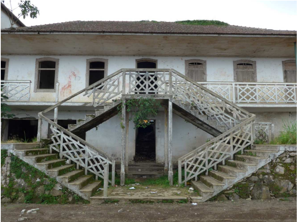
Fig. 31. Roça Monte Cafe, main plantation house, in a ruined state, 2015.
