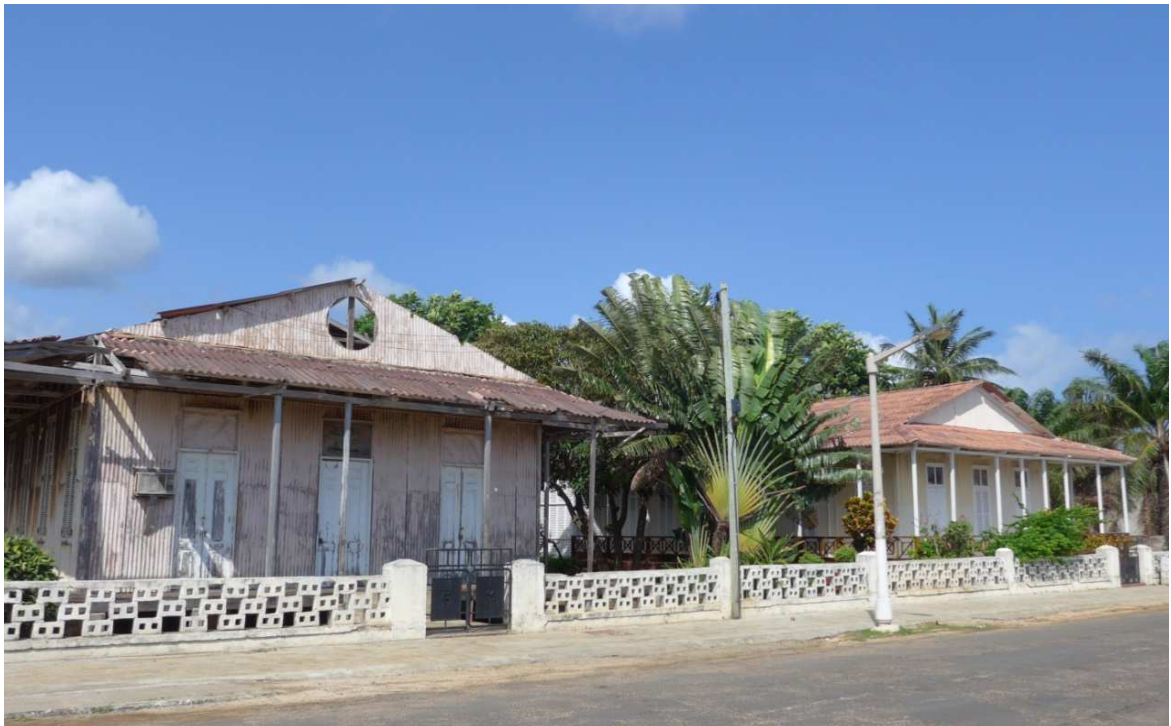
Fig. 84. Principal facades of two workers cottages at the S. Sebastião Maritime Station, 2015.
