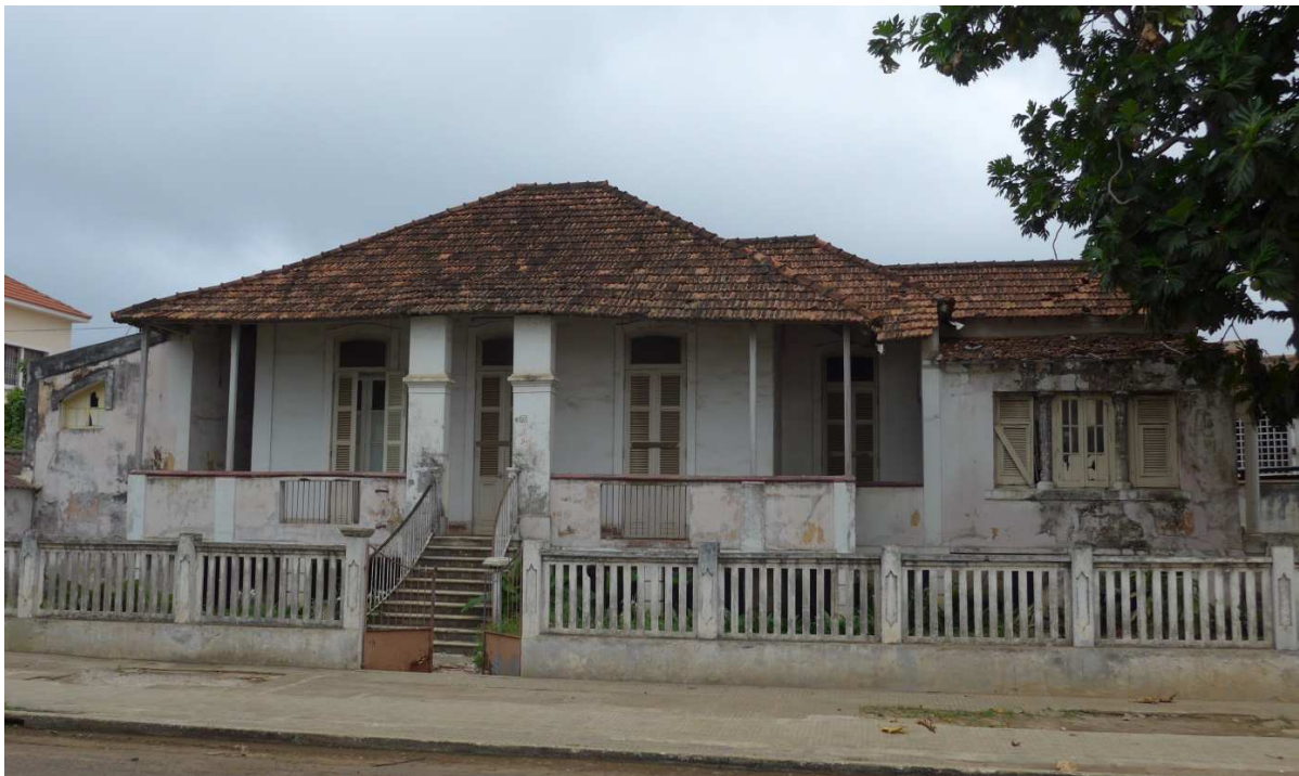
Fig. 81. Principal facade of station master's house at the S. Sebastião Maritime Station, 2015.
