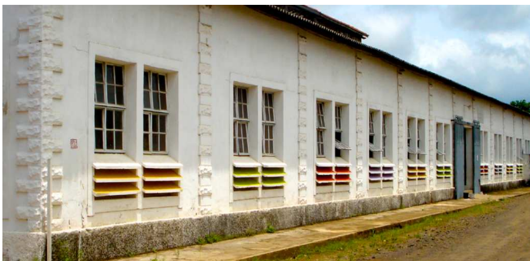
Fig. 77. The S. Sebastião Maritime Station: detail south facade of the railway workshop with square doorway, 2013.
