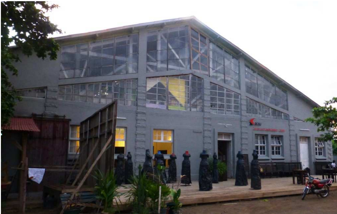
Figs. 74 and 75. The S. Sebastião Maritime Station: zooming in on the principal facades of the railway workshop, 2014.
