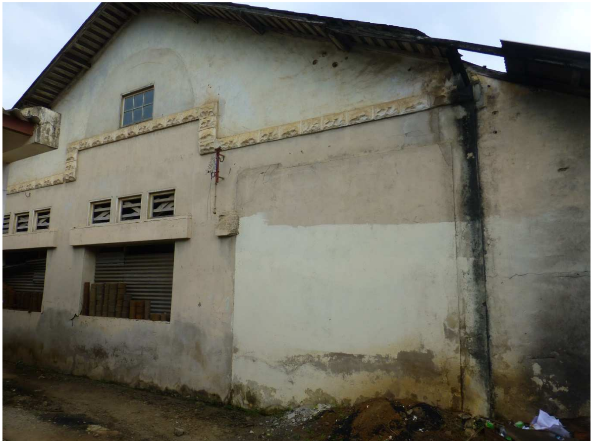
Figs. 102, 103. Side facades train shed anno 2016
