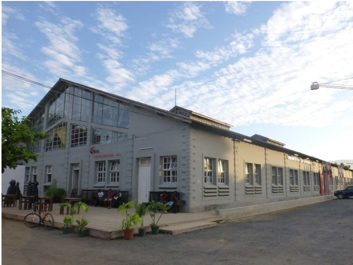
Fig. 73. The S. Sebastião Maritime Station: east and north facade of the railway workshop, 2014.
