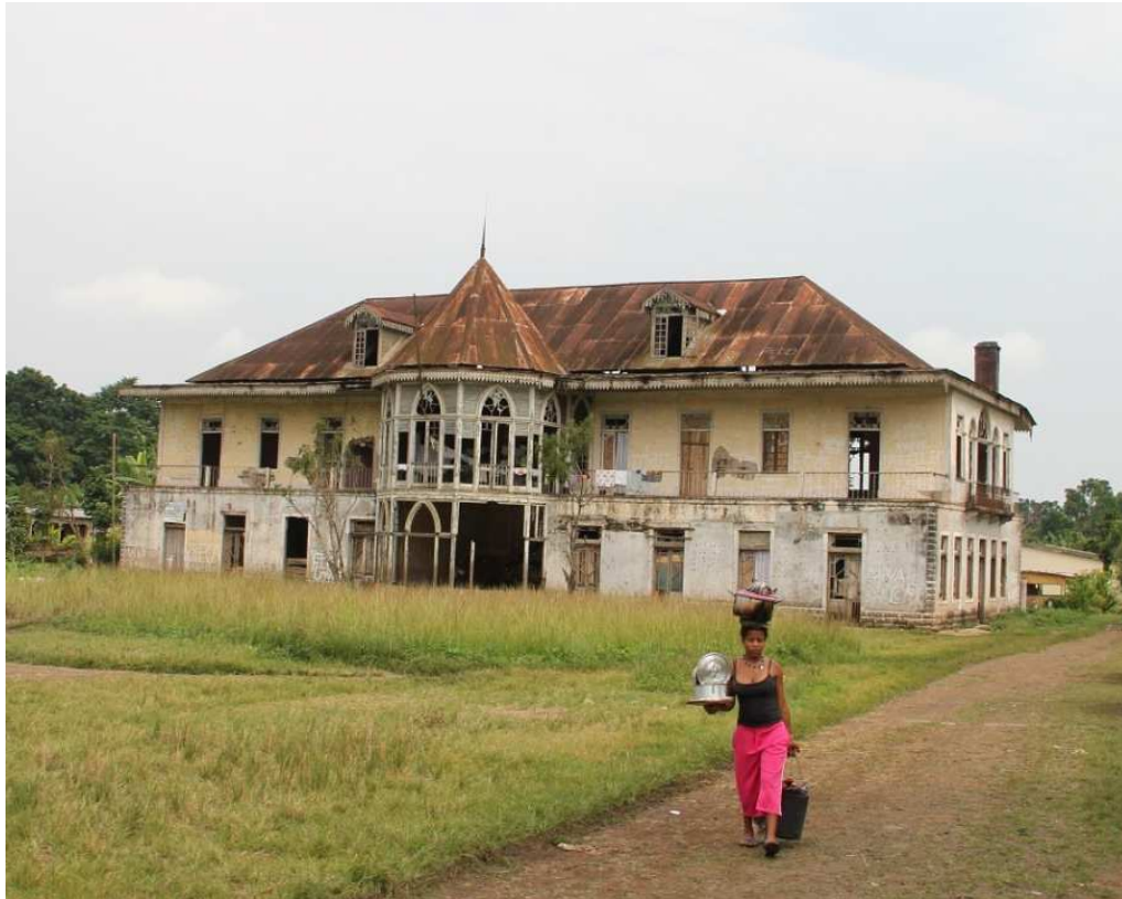
Fig. 5. Roça Boa Entrada. Note the crumbling, bow-fronted glass paneled facade, and fraying decorative wooden fretwork capping the main roof as well as the dormer windows (2013).
