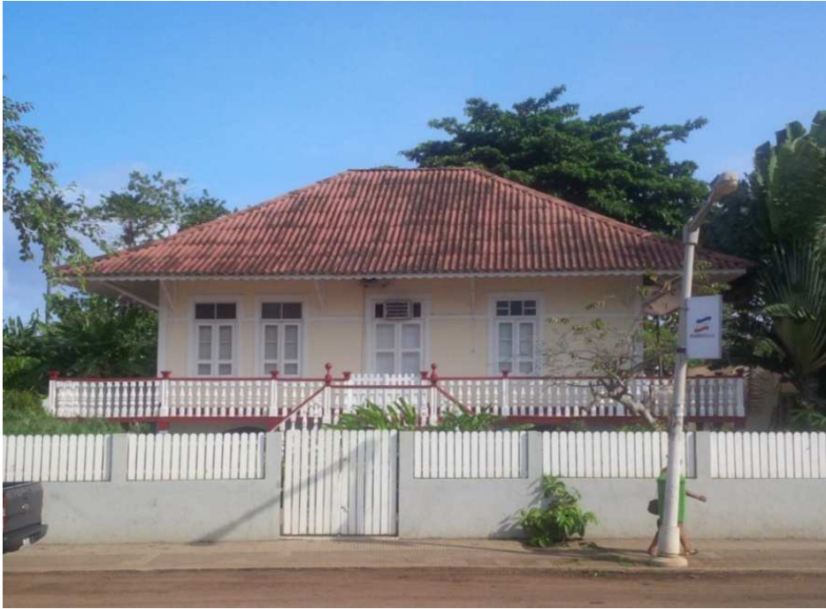
Fig. 36. Cottage São Tomé town dating back to 1910/1920 in 2015. Note the wraparound veranda, ornate balcony railing, louvered entrance door and louver shutters.
