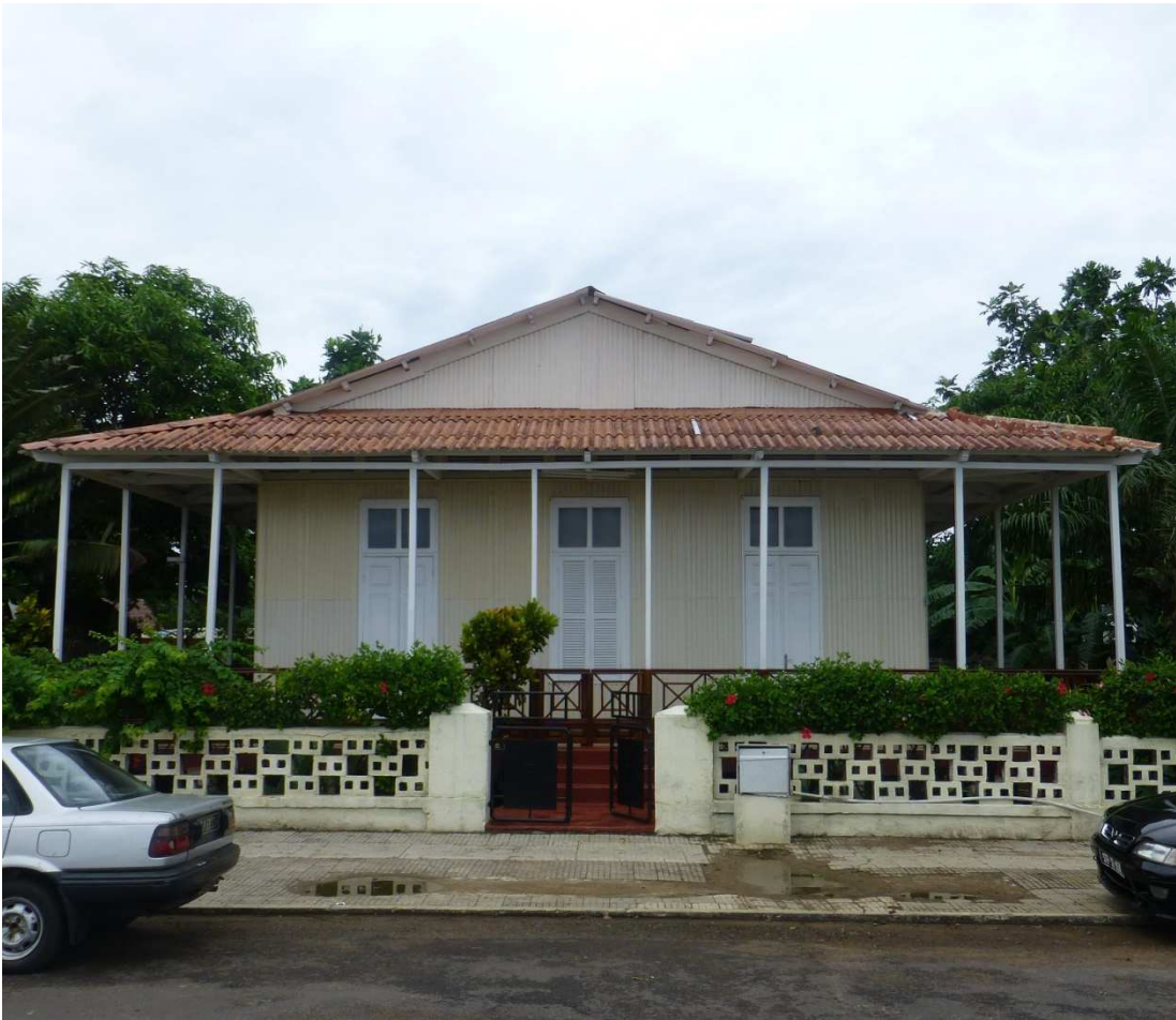
Fig 112. Facade of the adjacent sea fronting workers cottages, duly renovated, 2015.
