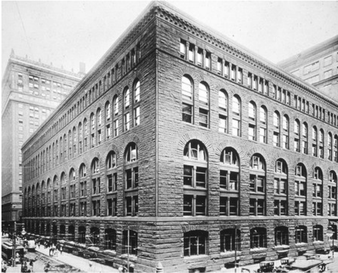
Fig 64. H.H. Richardson's Marshall Field Wholesale Store in Chicago (1885–1887), demolished 1930.
