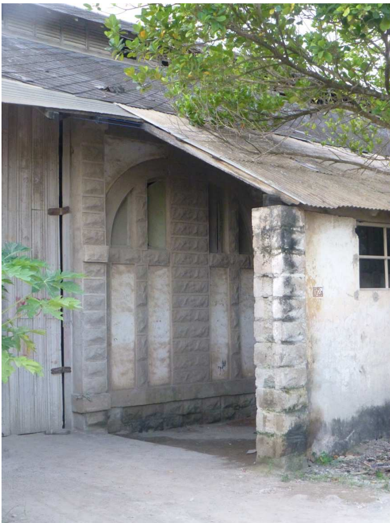
Figs. 104, 105. Elongated side facade train shed, anno 2016. Note the recent gate which insertion broke the original rhythm of rusticated arcades.
