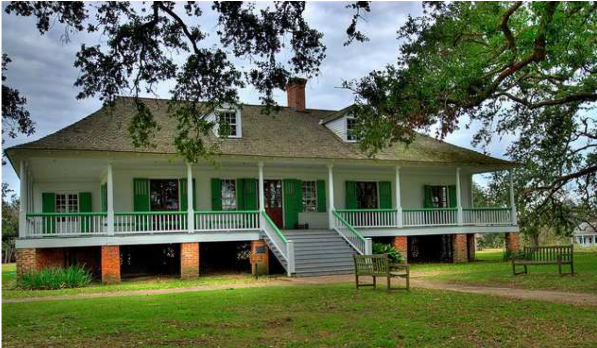
Fig. 19. Magnolia Mound plantation house, Baton Ville, Louisiana (current appearance dating back to the 1830s). Identifying features like being raised above grade, a (partial) wraparound veranda, & dual-pitched hipped roof were used at various STP plantation houses, like Roça Uba Bubu.
