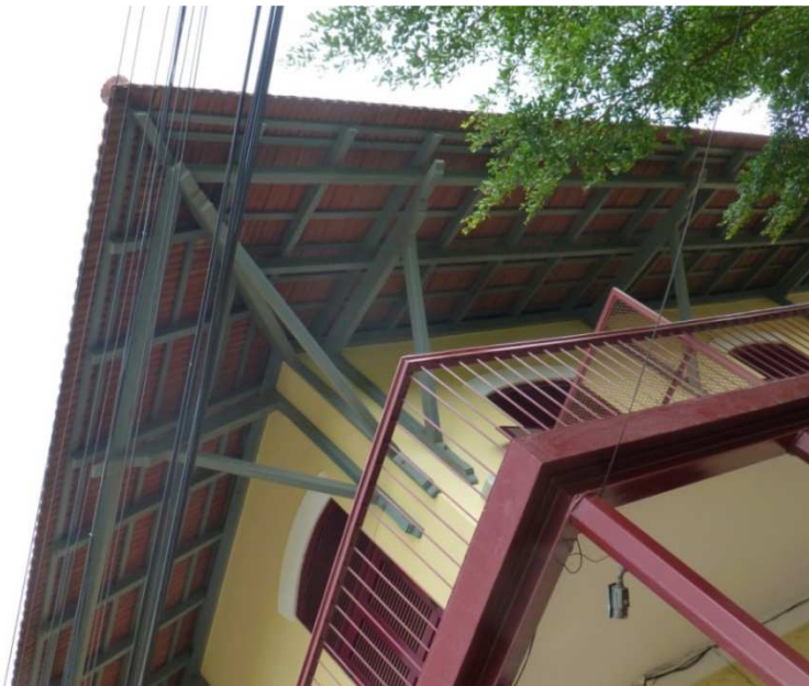
Fig. 55. Terminus station S. Sebastião, Detail of brackets supporting the hipped roof, 2014.
