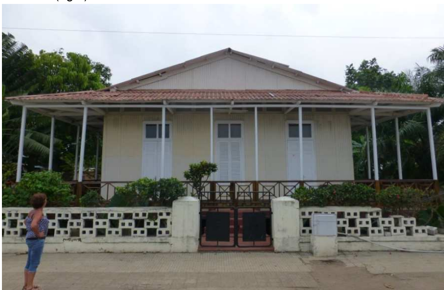
Fig. 87. Workers cottage the S. Sebastião Maritime Station, 2015..
