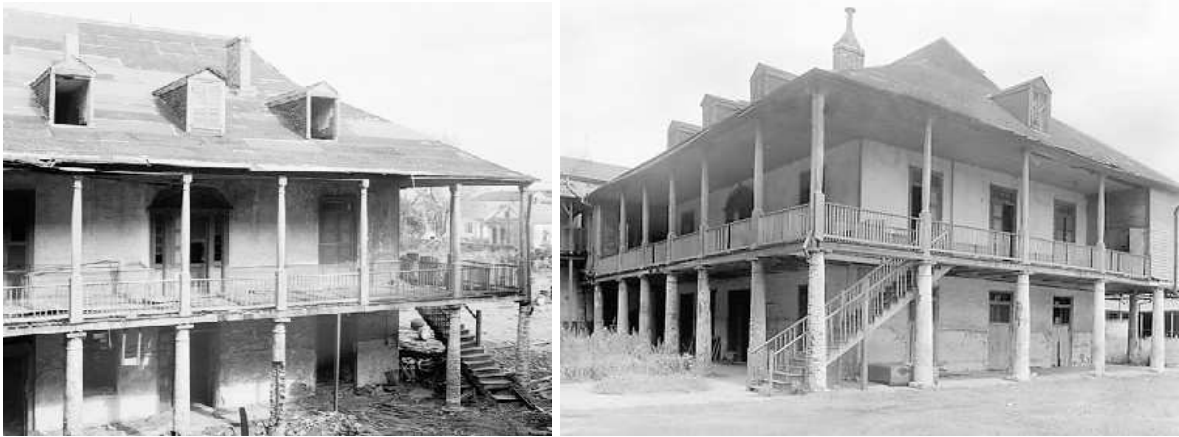
Fig. 18 A & B. The main plantation house of Olivier House, New Orleans, Louisiana. This building, dating back to 1820, was demolished in 1950. Identifying architectural features including wraparound verandas, brick columns & dual-pitched hipped roof were used at various STP plantation houses, like Roça Uba Bubu.
