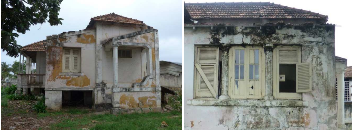
Figs. 82 and 83. Service wing at the station master's house at the S. Sebastião Maritime Station. Porte-cochere on the right, louvred window flanked by Tuscan columns on the left, 2015.
