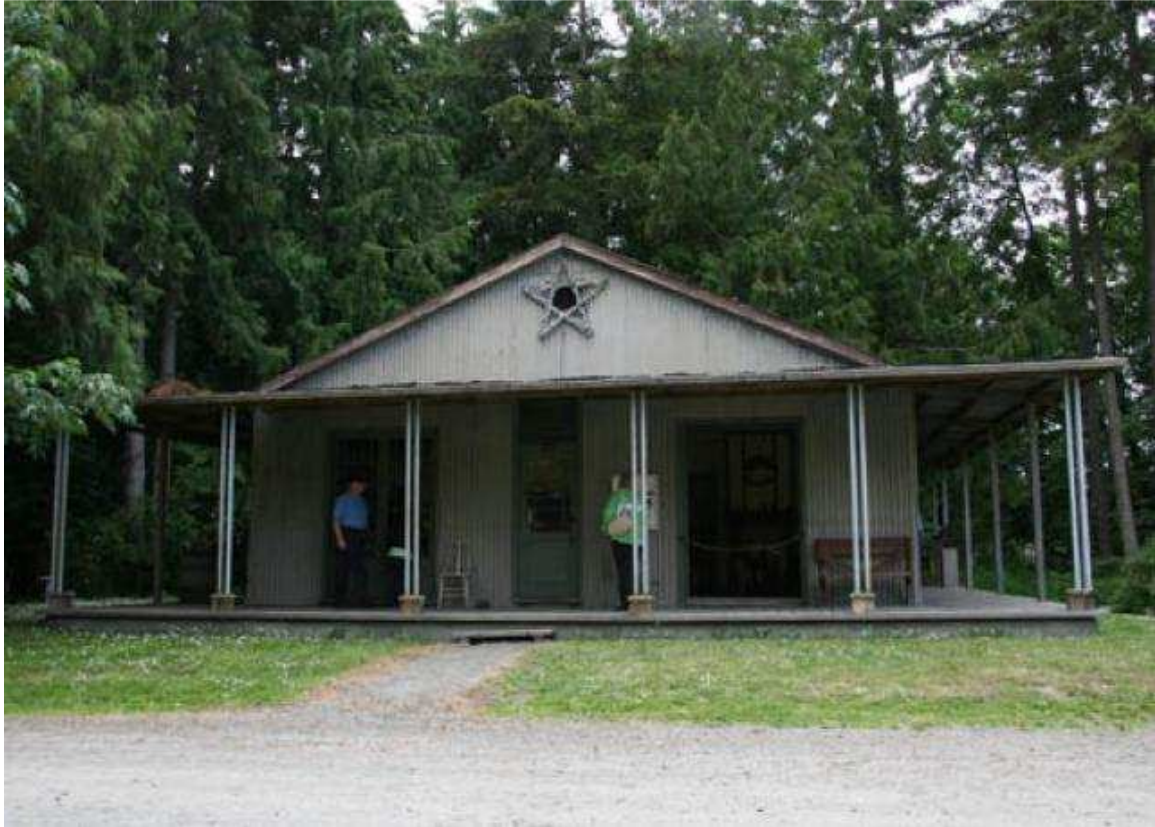
Fig.88. The Moody - Gosset House, a corrugated iron prefab house from 1859, British Columbia, Canada.
