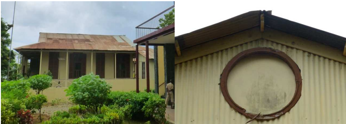
Figs. 92, 93. Long side of the 5th workers cottage, adjacent to the S. Sebastião station building on the left, round louvre opening main facade on the right, 2015.
