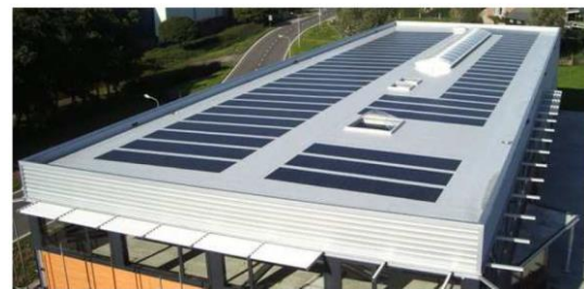
Figure 1-9: Examples of BIPV foil product (Alwitra GmbH & Co. (Jelle et al., 2012)) and embedded in a flat roof (WEKA DAKSYSTEMEN (Frontini et al., 2015)).
