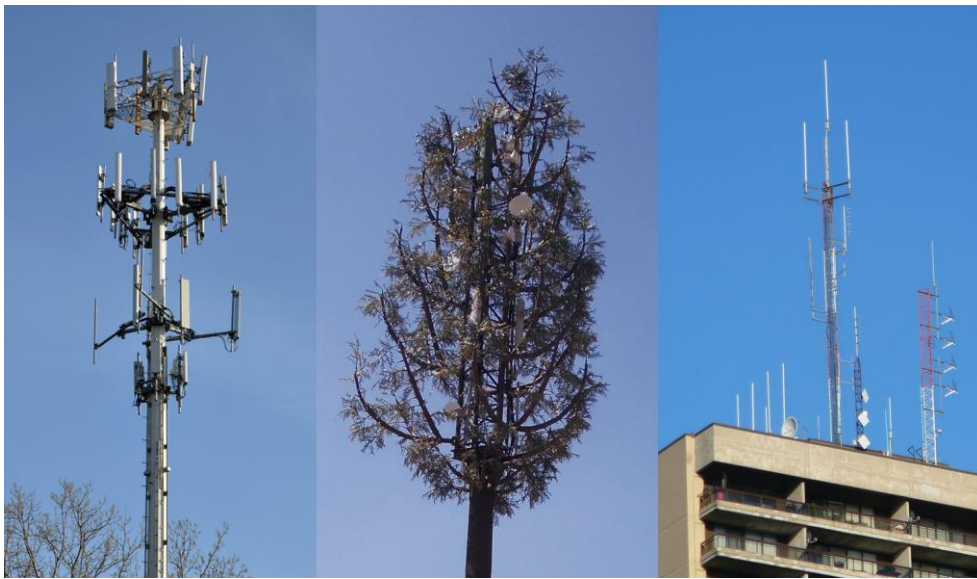
Figure 5.1, from left to right: a cell tower with antennas for various frequencies (2G/3G/4G), a camouflaged cell tower, and a cell tower located on top of a building.
