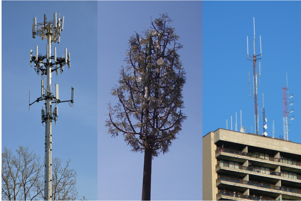
FIGURE 5.1: From left to right: a cell tower with antennas for various frequencies (2G/3G/4G), a camouflaged cell tower, and a cell tower located on top of a building.
