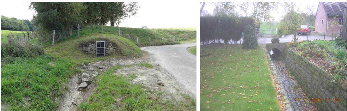
Figure A-5: A closing valve at a buffer outlet (left) and a culvert incorporated in the landscape (right).
