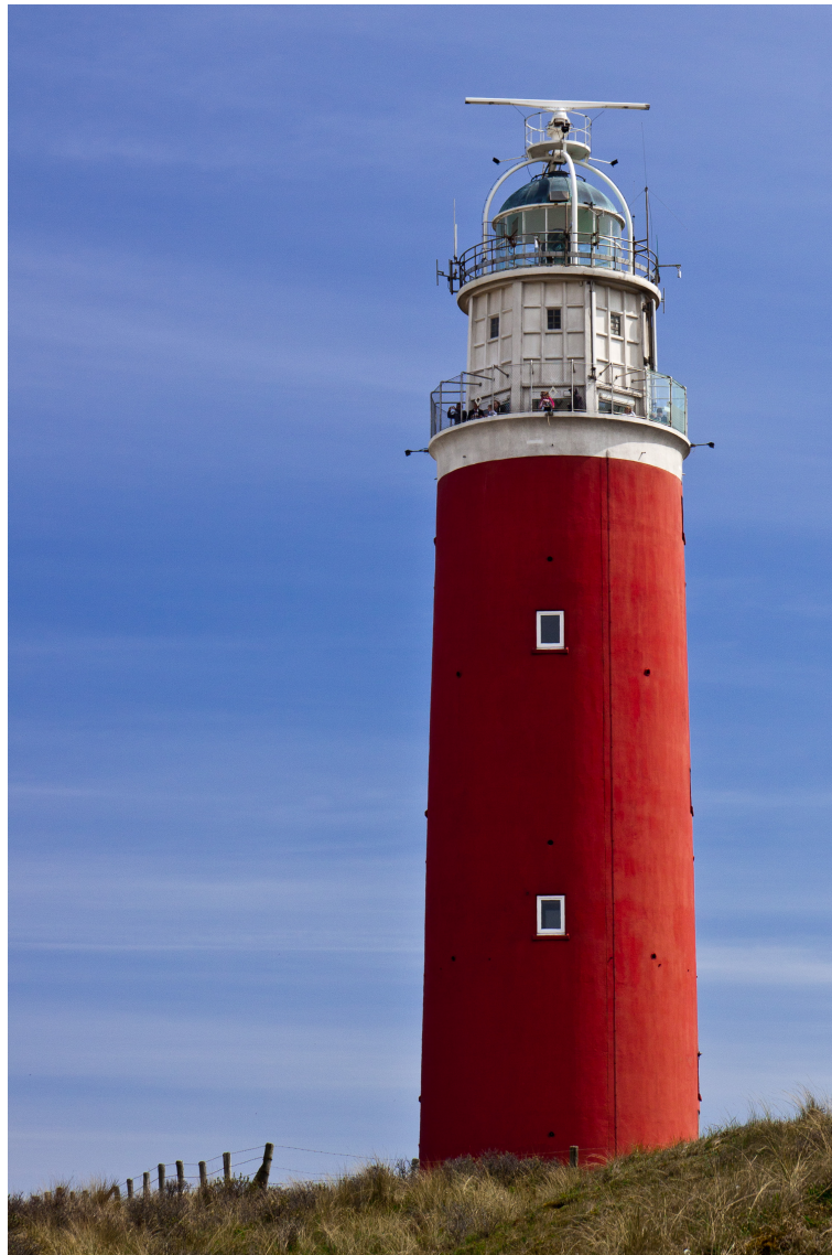
Figure 2.1: The Eierland lighthouse on Texel with on top a characteristic coastal radar antenna and on the left at the second ring an AIS antenna. 6
