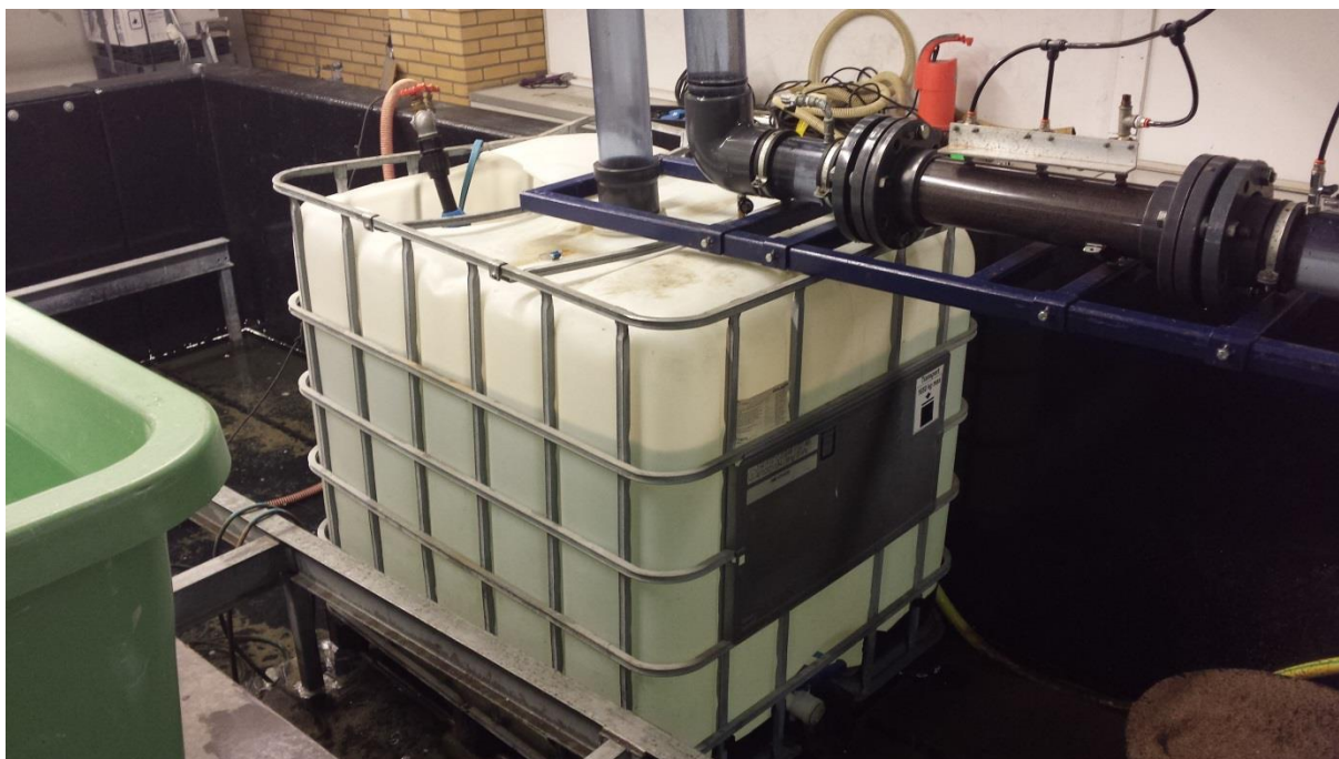
Figure A-4: Reservoir which is parts of the setup. Supplies water to the rest of the setup and functions as water catchment for the water leaving the setup.
