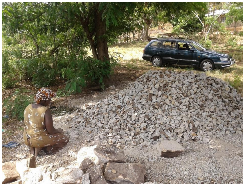
An aggregate producer at work
