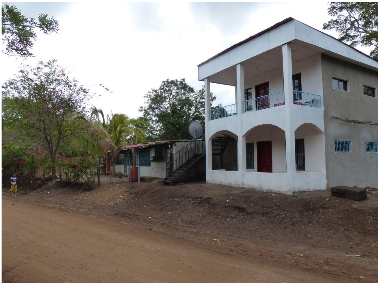
Figure 15: The homestay on the left was able to invest in the construction right, able to host four tourists instead of one
