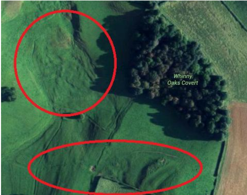
Figure 5-35: Landslide at Whinny Oaks Covert
