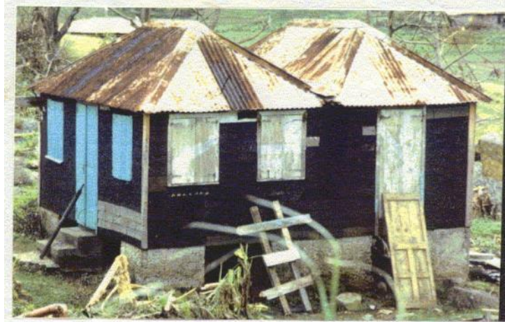
Figure 2-4 Thanks to a favorable geometry and roof shape, this building survived the hurricane Hugo, source: (Gibbs, 2001)
