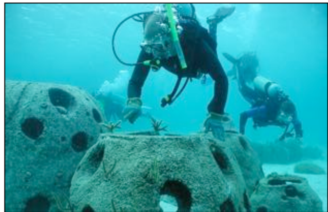
Figure 4.7 Concrete 'balls' as artificial reefs. Source: Muscat Daily
