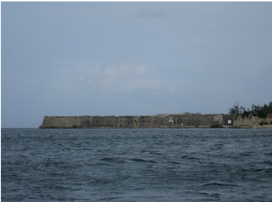
Fig. 3.3: The western front of the São Sebastião fortress as seen from the bay of Mossuril.
