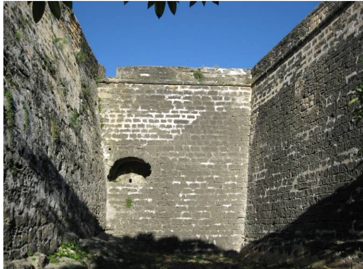
Fig. 3.6: Former main gate of the fort, located within the southern curtain at the point where the two wall section meet. Fig. 3.7: The retired flank of the Santa Bárbara bastion, showing the traces of what would have been a vaulted opening.
