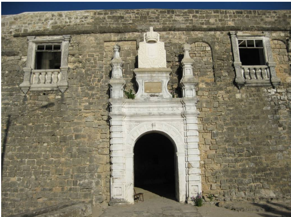
Fig. 3.5: Main gate of the fortress, located within the western curtain. Above the decorated façade traces of earlier windows are still visible.
