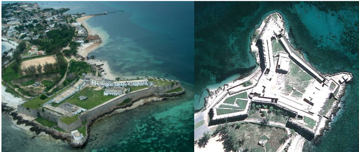
Fig. 3.1 & 3. 2: Areal views of the São Sebastião fortress at present. From above the traces of older building phases are clearly visible.
