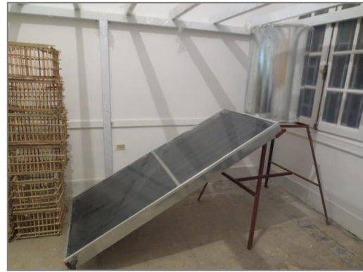
Figure 12. The final DIY solar water heater
