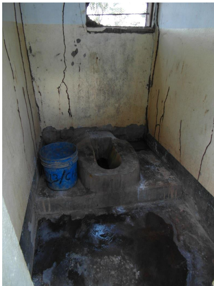
Figure 6.2 Girls' toilet at secondary school Magu, Tanzania
