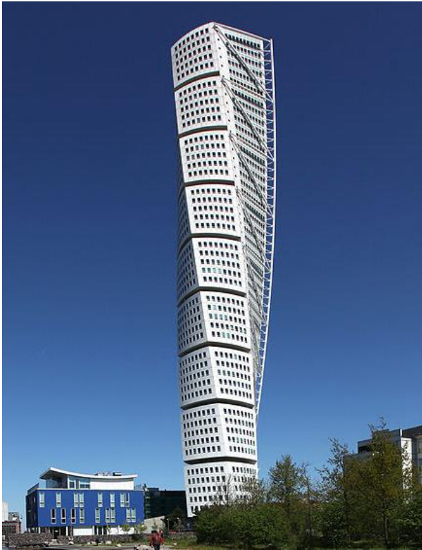
Figure 6.3: Turning Torso: iconic image of the city of Malmö
