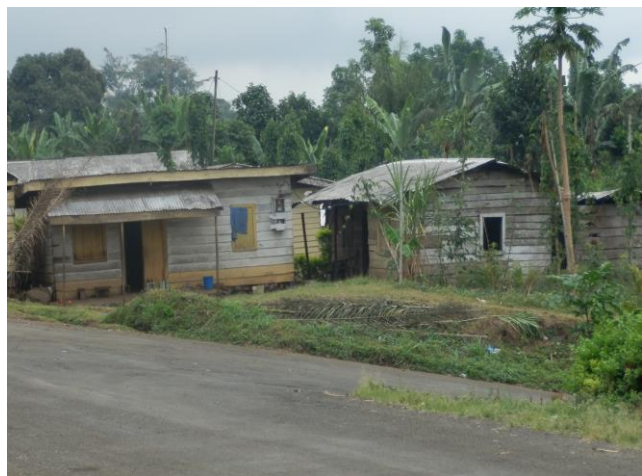
Picture 4.4: Houses with wooden walls in Bonakanda in the mountainous area, South West Region, 2014.
