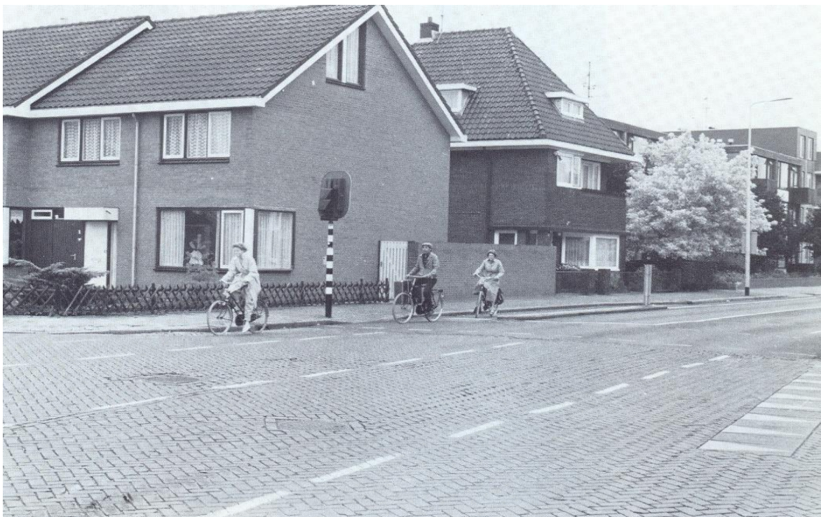
Figure A5.17: The same corner in 1986. Photo: T. Wiegman
