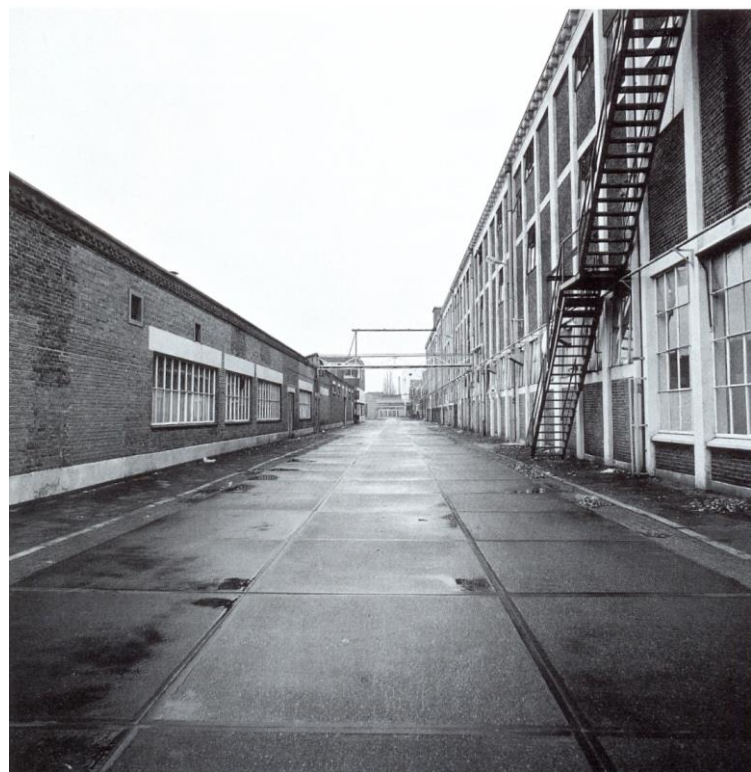
Figure 4.12: The Bamshoeve factory halls in the 1990s Photo: Johan Ghijssels
