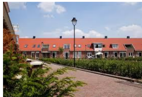
Figure 5.2: Houses in Roombeekhofje Photo: USHI Kenniscentrum Bouwen
