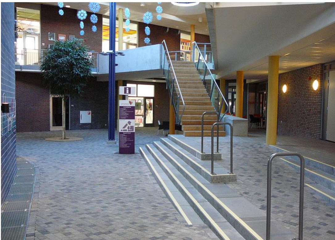
Figure A4.2: Interior of Prismare Photo: Municipality of Enschede
