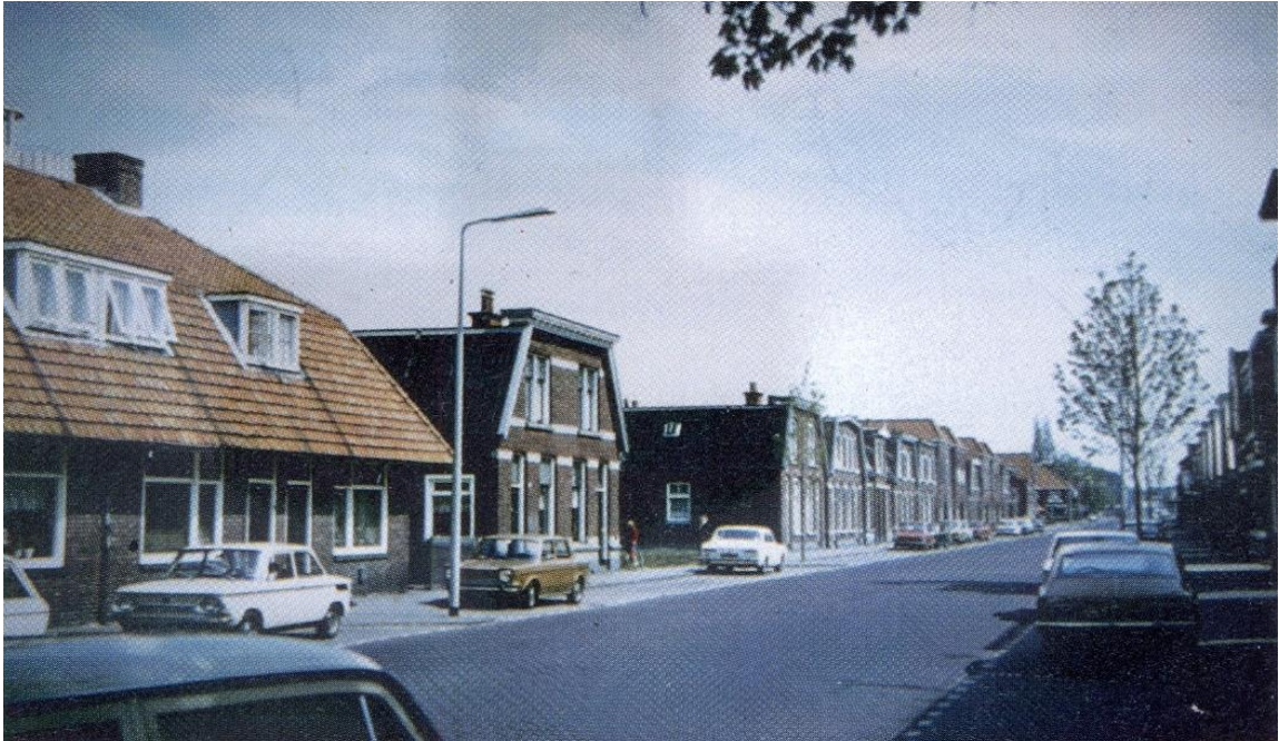
Figure A5.7: The Roomweg in the 1950s Photo: T. Wiegman
