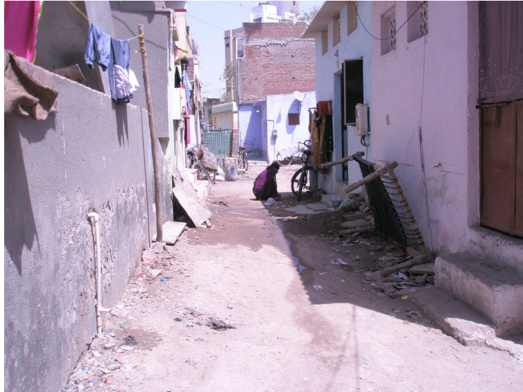
Figure 3. 6. High thresholds to keep water out during the monsoon.
