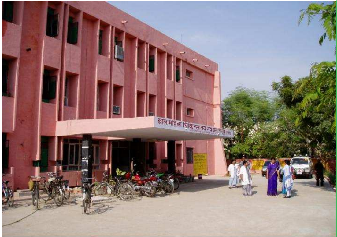
Aliganj Bal Mahila Chikitsalaya evam Prasuti Grah (Maternity Home) after renovations and repairs.
