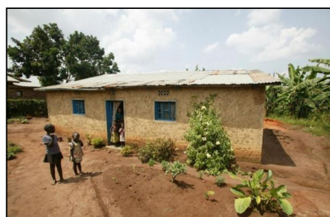
Illustration 5.2: A common shelter: made of corrugated iron and mud
