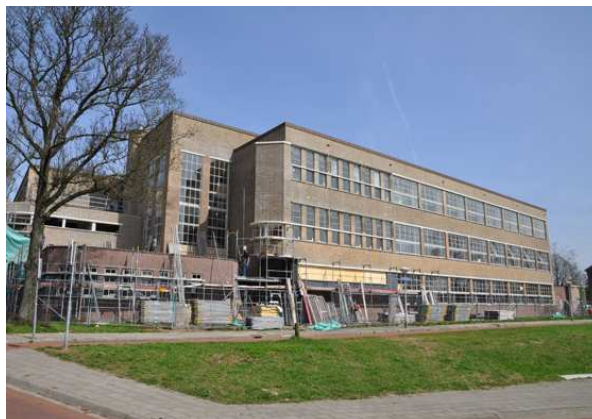
Picture 7. Ambachtsschool under construction.
