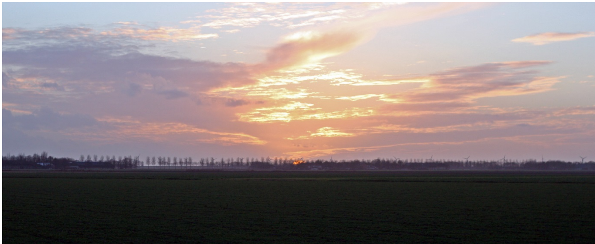
Figure 5.7 Current Westermeer binnendijk wind farm
