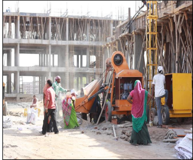
Picture 4.15. Construction site at Madhav Homes in Vastral
