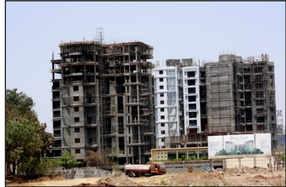
Picture 4.7. Construction Site Golden Trellis
