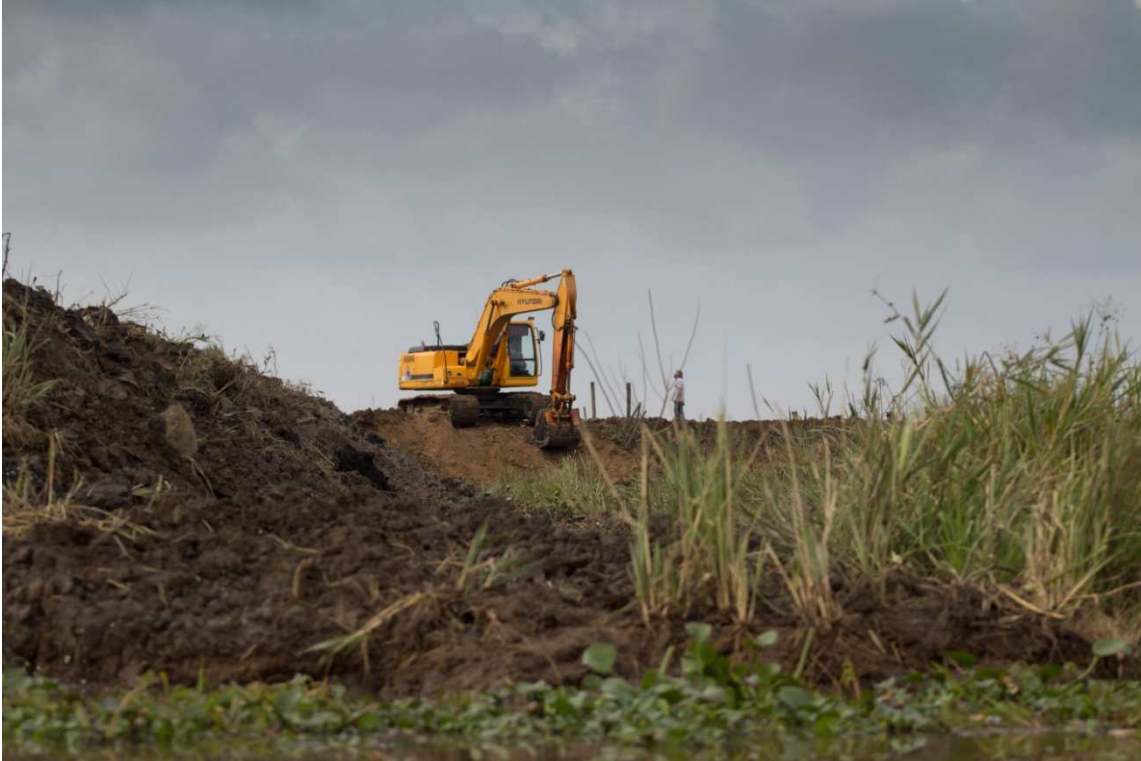
Figure 29 – Embankment works in the Baradero Delta region (own source)
