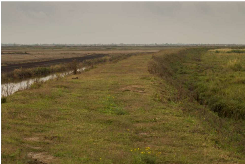
Figure 27 - Embankment in the Baradero Islands (own source)
