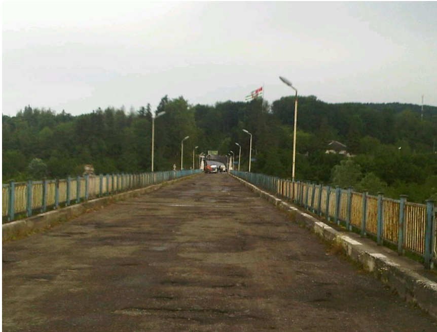
Figure 4: The Inguri Bridge while heading towards the Abkhazian border crossing.
