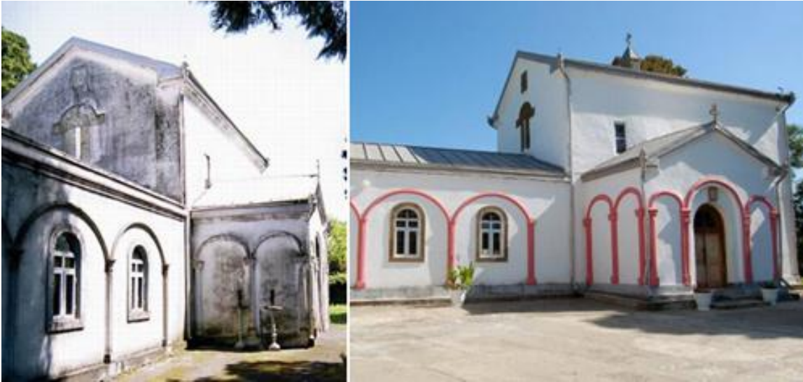
Figure 1: On the left side a picture of the Ilori Church before renovation, on the right side the Ilori Church after renovation.
