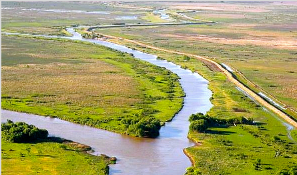
Figure 9: Dikes constructed by Pazzaglia Brothers S.A. (source: Fundación Proteger, 2008)
