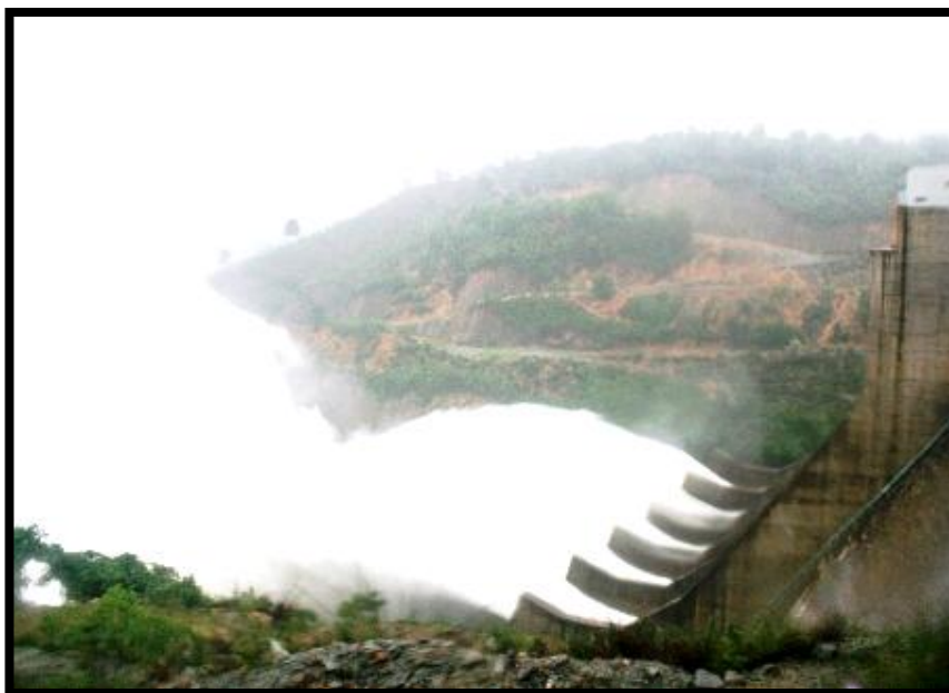
Figure 6: Binh Dien hydropower dam
