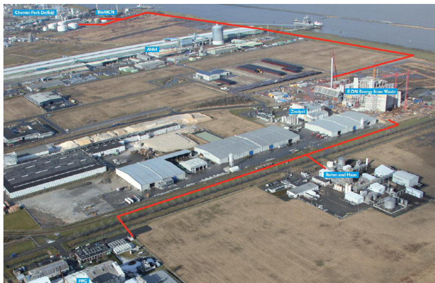
Figure 17: Steam pipe Delfzijl (Agentschap NL, 2011a)
