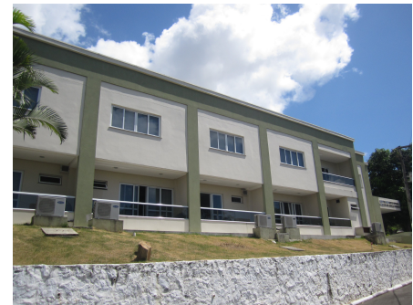
The CPN from the side. On the ground floor, 6 'p.p.p' rooms with varanda. Upstairs, offices and a memorial. Picture taken by author
