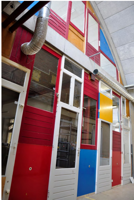
Figure 3.3 – wall made of secondary doors and windows (source: Slager and van der Veen, 2012)
