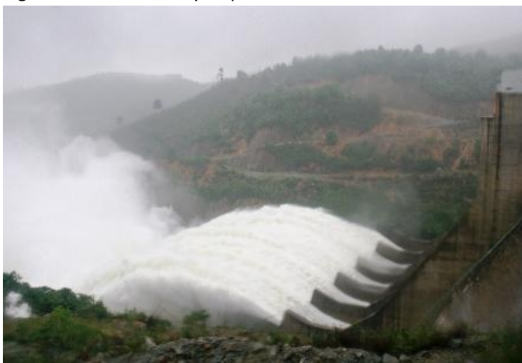
Figure 8.1: Binh Dien hydropower dam
