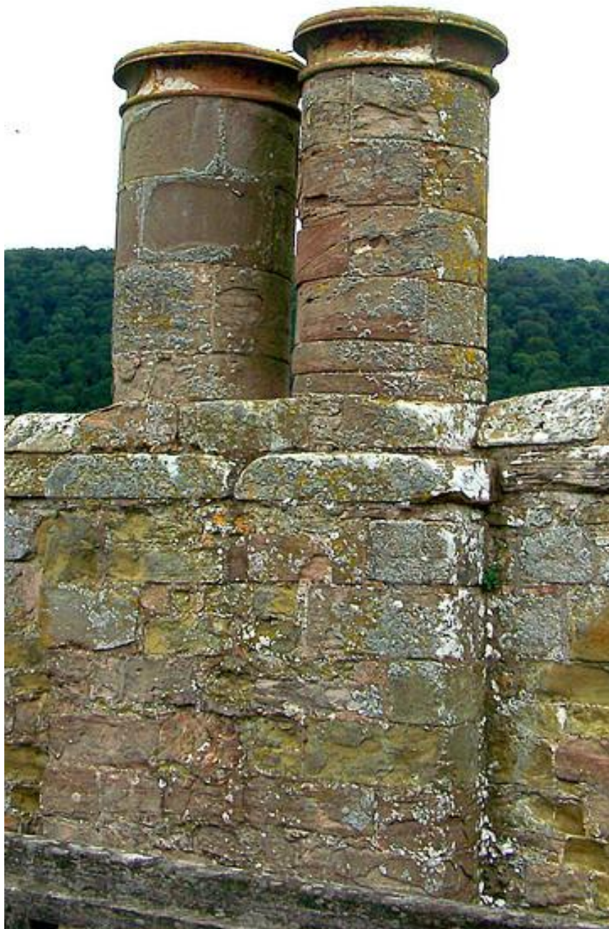
Dubbele schoorsteen, Stokesay Castle, Shropshire, ca. 1290.
