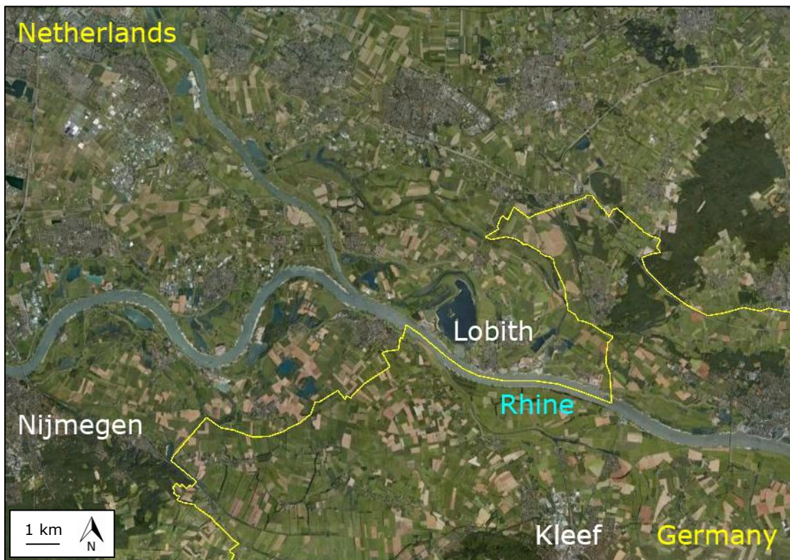
Figure 1: The Rhine where it enters the Netherlands at Lobith (Google Earth, 2013)
